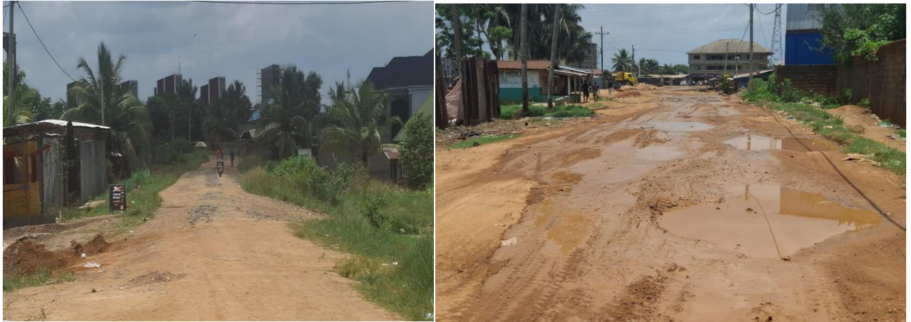
Figure 2: Partial View of Segment 2 of the Project Corridor
